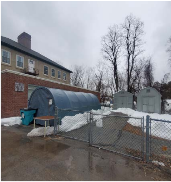
South side, storage units
