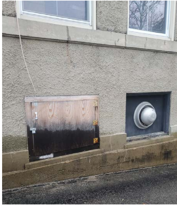
West side, Uninsulated side hatch
