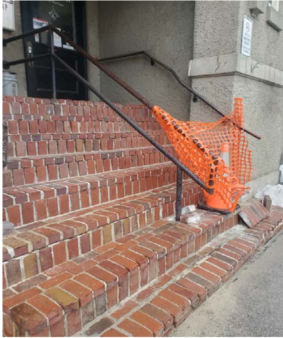
North side, Front Entry Stairs
