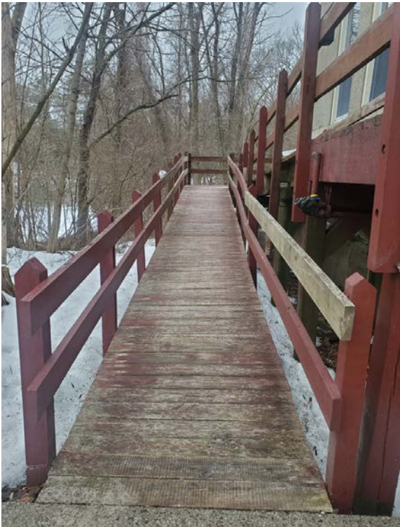
East side, Wooden ramp
